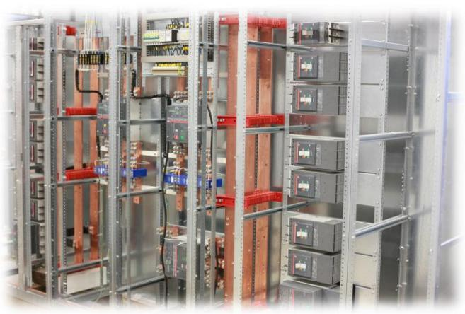
Switchgear Motor Controls Standoff Insulators Control System Components Circuit Breakers Arc Chutes
